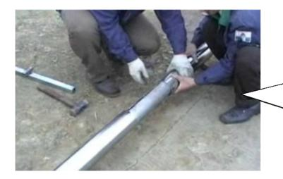
One piece pole is inserted In the second pole
